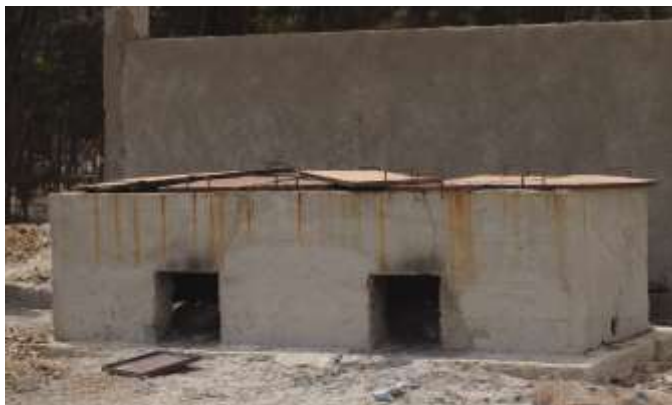
Figure 5: A double Parpaing oven with steel lids on top. (Photo from JV, 9/20/2020)
